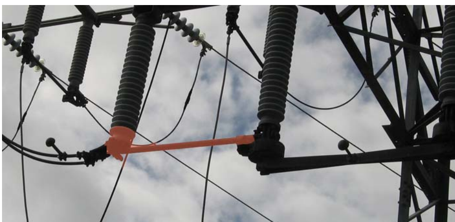
Example of a closed disconnect switch.
